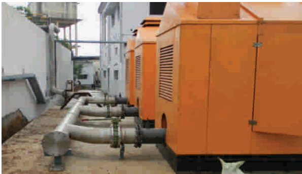
Fig: Air blowers for Aeration
