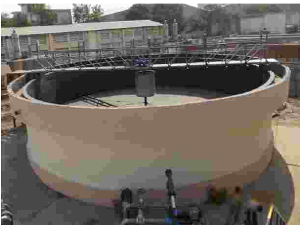
Fig: Secondary clarifier system
