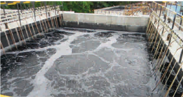
Fig: Aeration tank (aerobic biodegradation)
