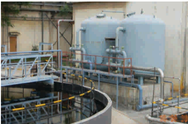
Fig: Tertiary system (TC/ CCT/ PSF/ ACF)
